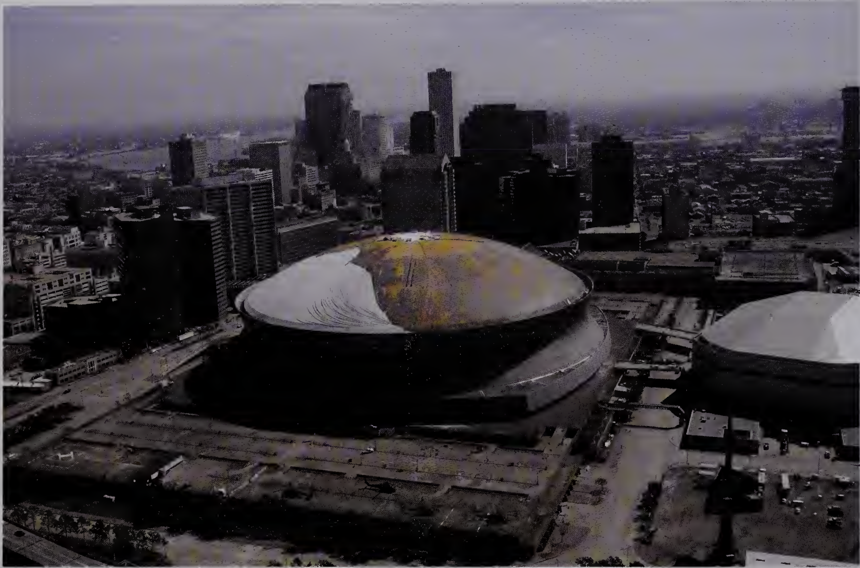
The Superdome with its storm-damaged roof
